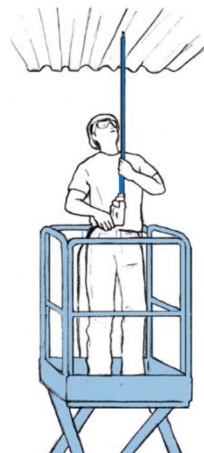
Drill-bit extension shaft with plastic sleeve; work platform.
